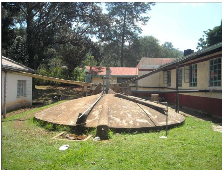
Figure 1. Cistern with collecting troughs for capturing and storing rainwater.
